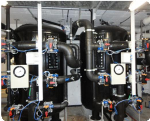
Fig. 2: Two identical quick filters
