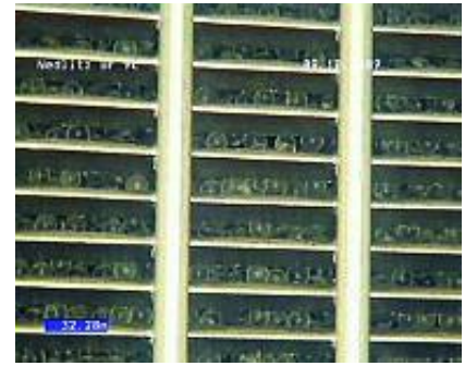
img. 4 Well filled with bulk glass balls and wound wire filter
